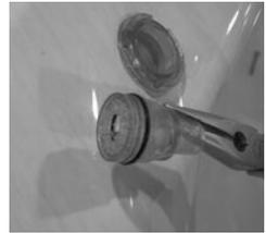
4. Clean plastic diffuser at the back of the Jet insert or Laminar Flow Jet Assembly so all holes are free of debris.
