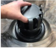
*Pull Up to Remove Floater Assembly*
